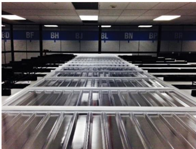
Melt away ceiling panel installation
