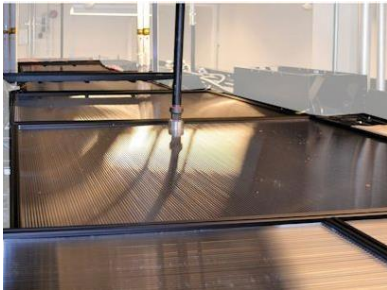
The fire suppression system was brought down below the rigid ceiling
