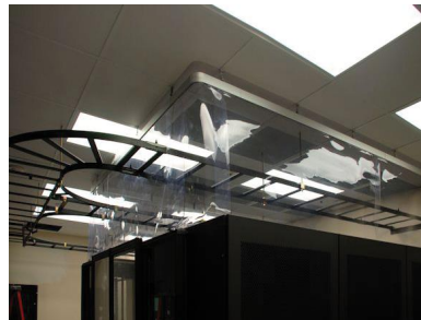
Vinyl Curtain cut around ladder rack
